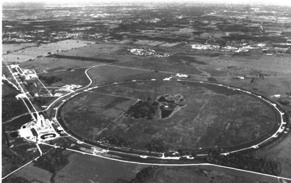
A state-of-the art version of a proton synchrotron. Here at Fermilab protons will be accelerated to an energy close to 1 TeV in a 6562-foot-diameter ring of superconducting magnets. Wilson Hall, headquarters of the laboratory and a fitting monument to a master accelerator builder, appears at the lower left. (Photo courtesy of Fermi National Accelerator Laboratory.)
